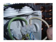
cal box of the fan unit and connect the leads into the tree in the upper right side of the box. The ground wire (green) needs to go in the center terminal, but past the wires' placement doesn't matter - that is to say that whether the black or white lead goes on the left or right does not matter. Presto, you're finished - unless you want to add on an:
