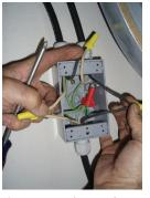
should connect to the black lead which comes down from the temp controller. The white lead from the wall should connect to the white lead from the fan unit. Finally, connect the white lead from the temp controller to the black lead from the fan unit to complete the circuit.
